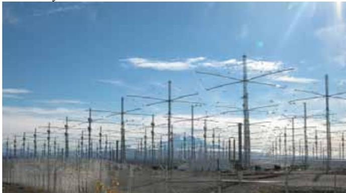
Comprised of 180 antennae approximately 22 metres tall, which are linked together to function as one, HAARP can direct a powerful energy beam into the ionosphere, a region of the upper atmosphere.
