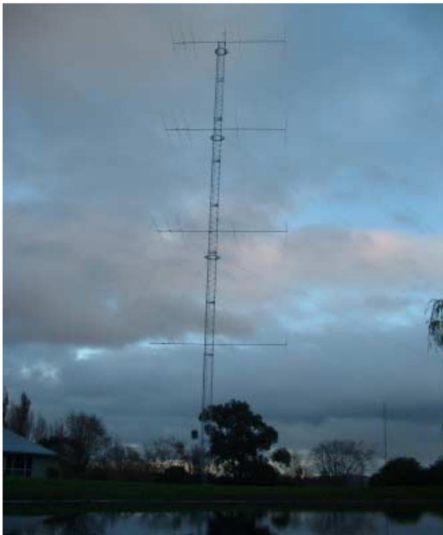
At 200 feet high (60 metres) **Ian VK3MO** has perhaps the best amateur tower in Australia? And forget about rotating the beams.....all four of them.....the actual tower is able to be rotated!!
