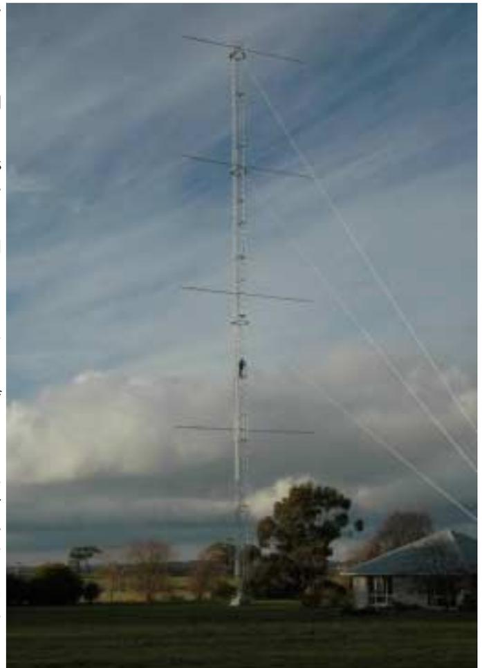
All the tower sections have an 80mm face, but the leg diameters reduce. The lower sections use 50mm solid bar and reduce gradually to 37mm diameter on the upper sections)
